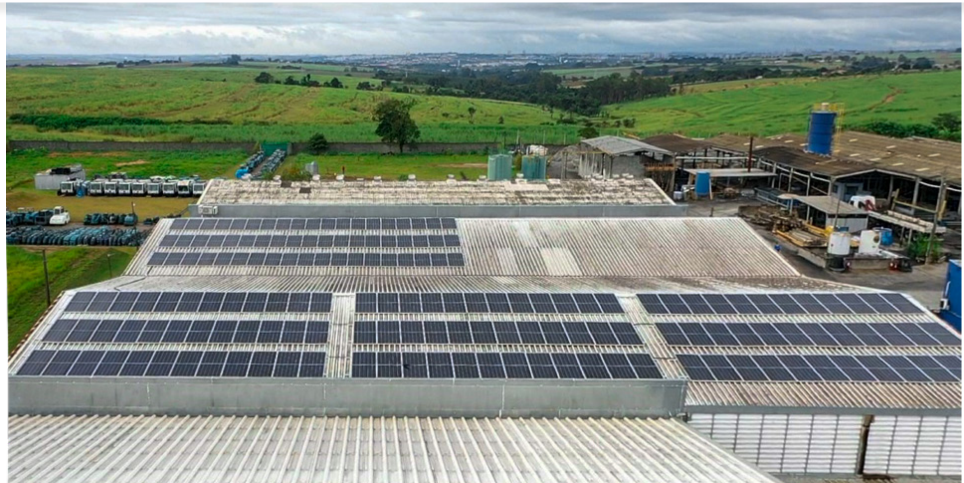
Solar panels on Limeira, Brazil, plant
